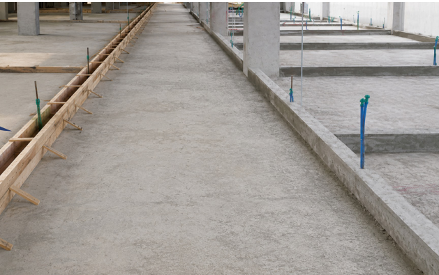
Conventional Reinforced Concrete Waterproof Curb
