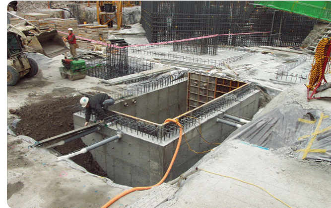
Difficult to install drainage pipes and high risk of pipe damage
