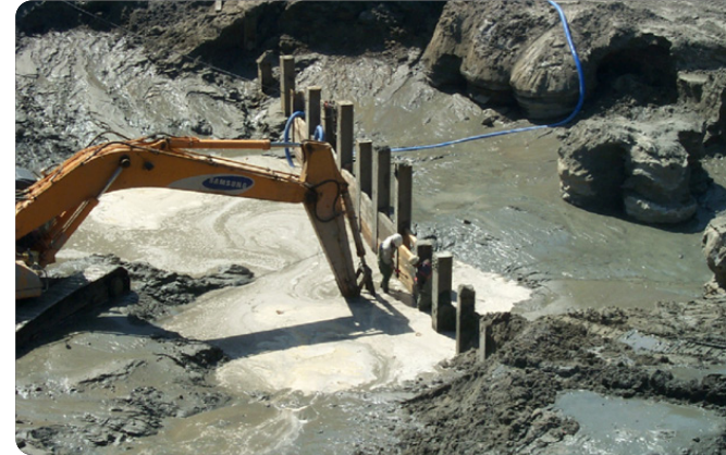
Groundwater inflow degrades concrete quality
