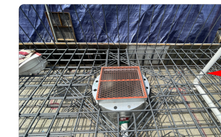
4. Fix with Top rebar
