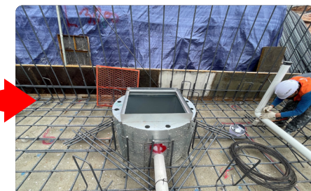
3. Fix with Bottom rebar
