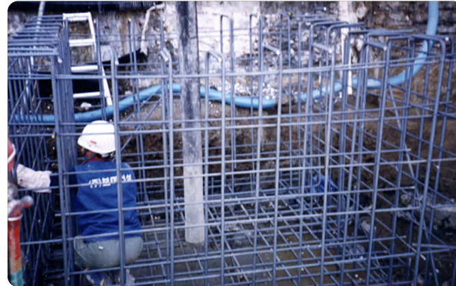
High rebar density increases construction difficulty
