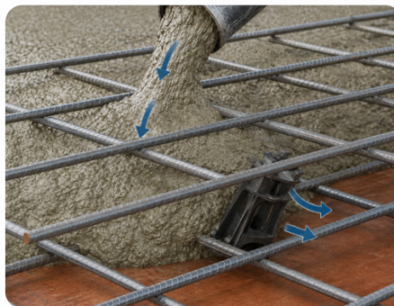
Displacement during concrete pouring
